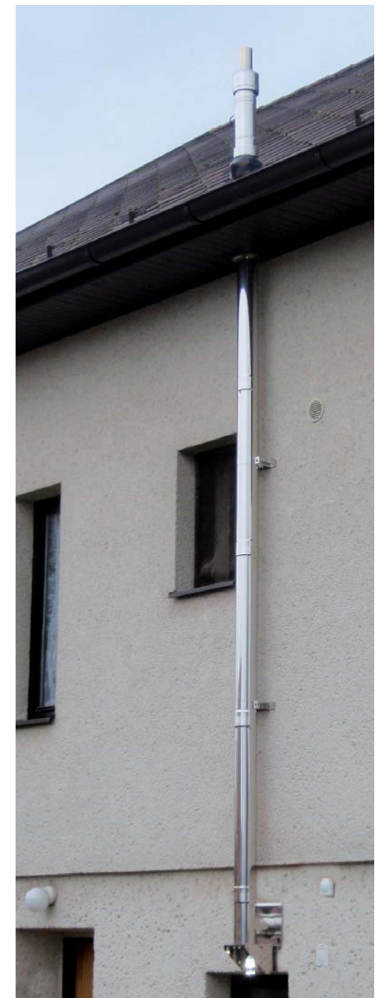
External flue gas discharge using concentric elbow and combustion air intake through vertical terminal
