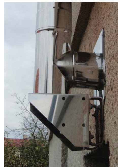
External flue gas discharge using elbow w. support and combustion air intake
